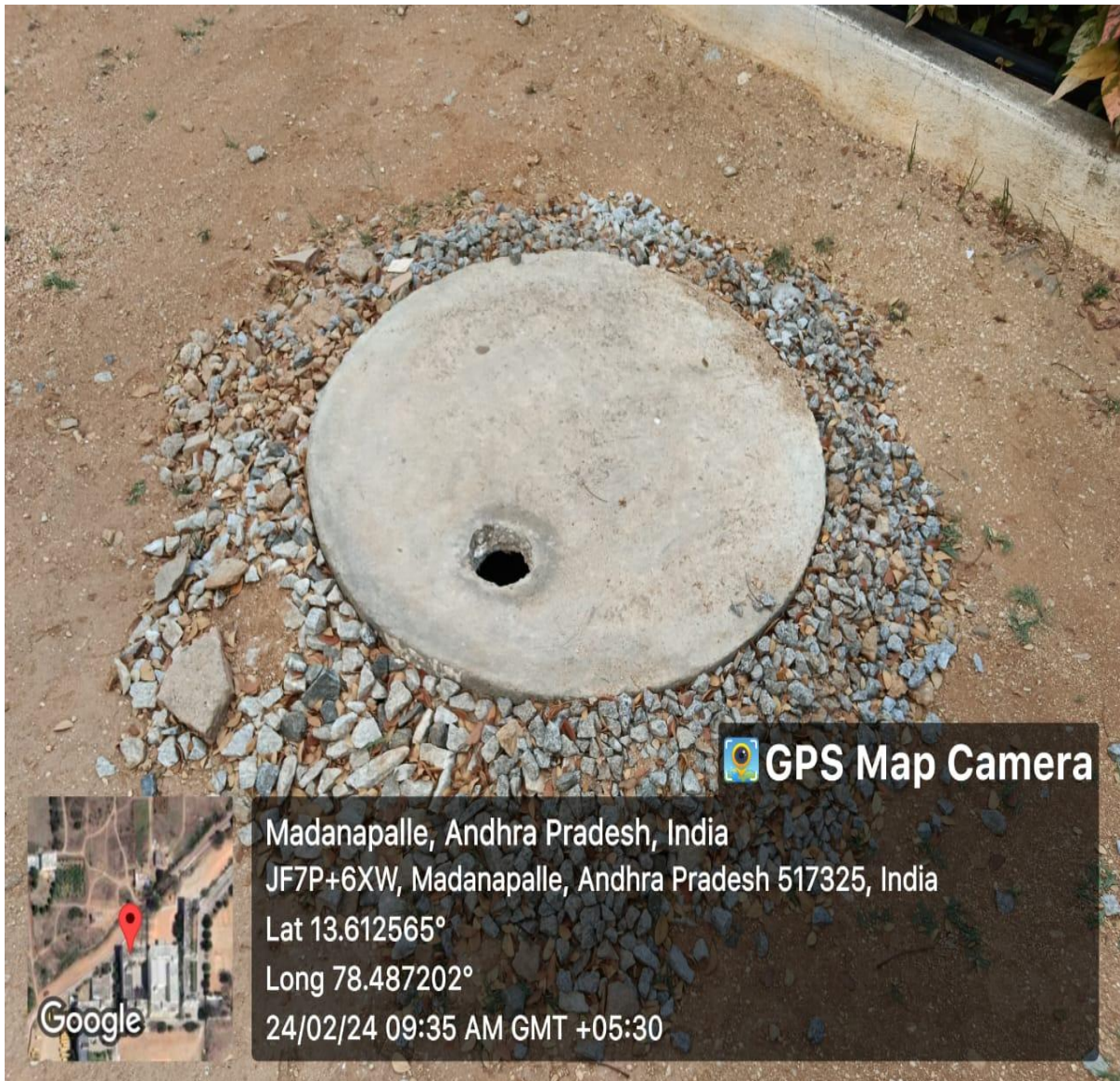
Rain water harvesting pit
